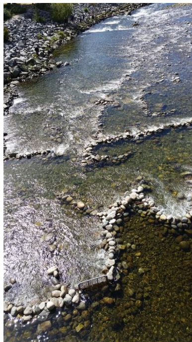
Fig. 6. Stone weir at the mouth of the Capilano River, Vancouver, BC. Photo taken by me.
