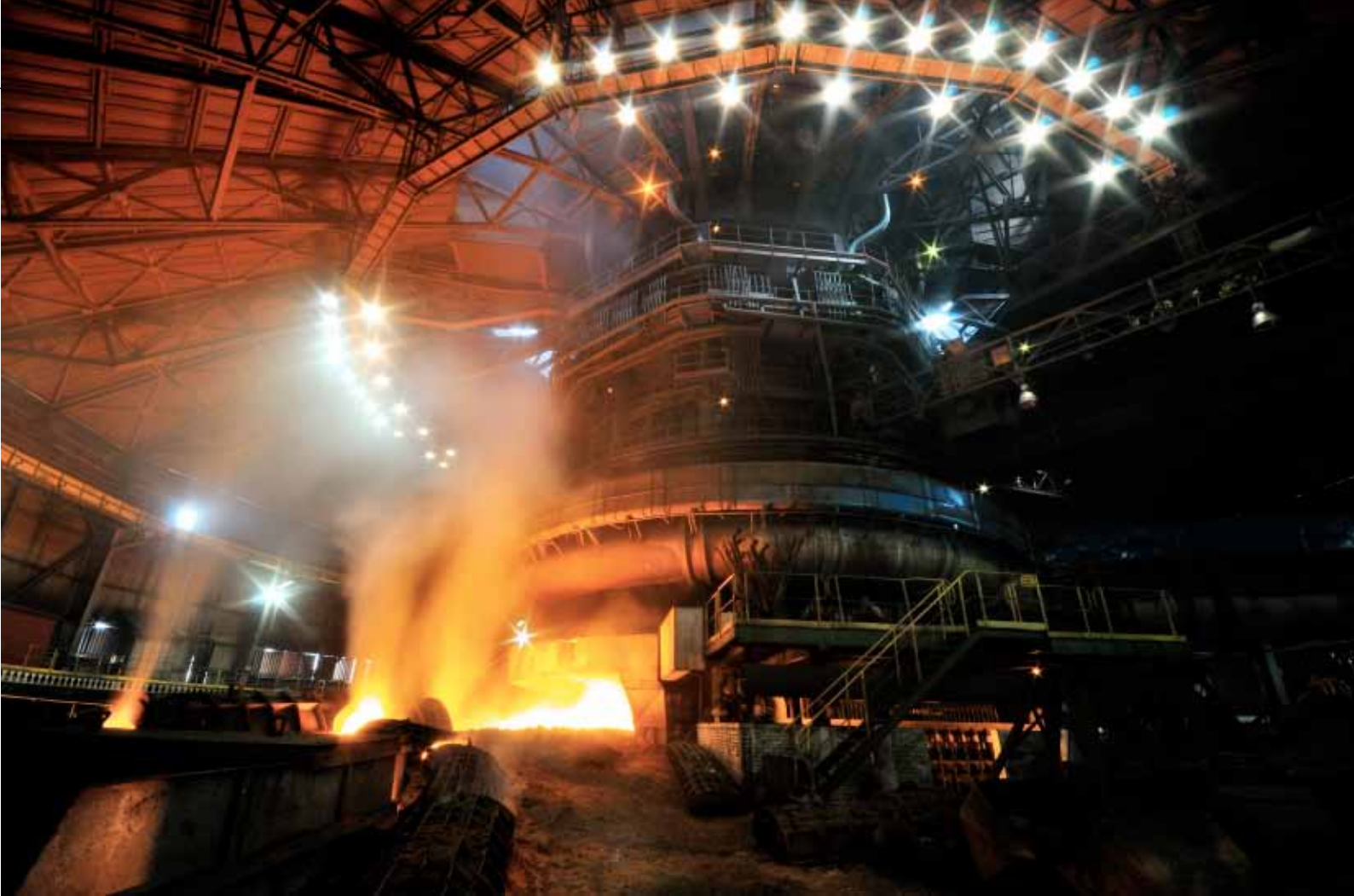
Wielki piec. Fot. ArcelorMittal Poland S.A.
