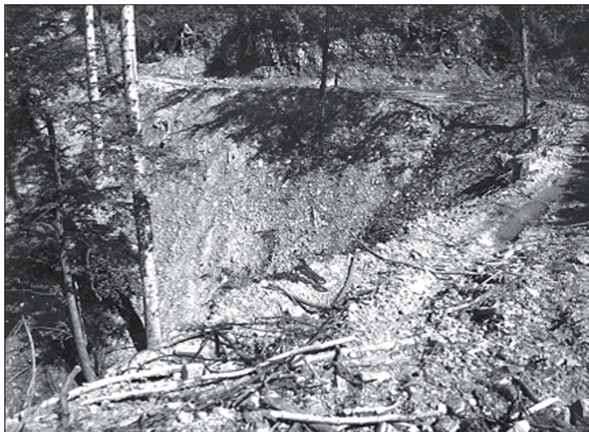
Phot. 2. Forest road damaged by tractors (phot. by L. Buzek)
