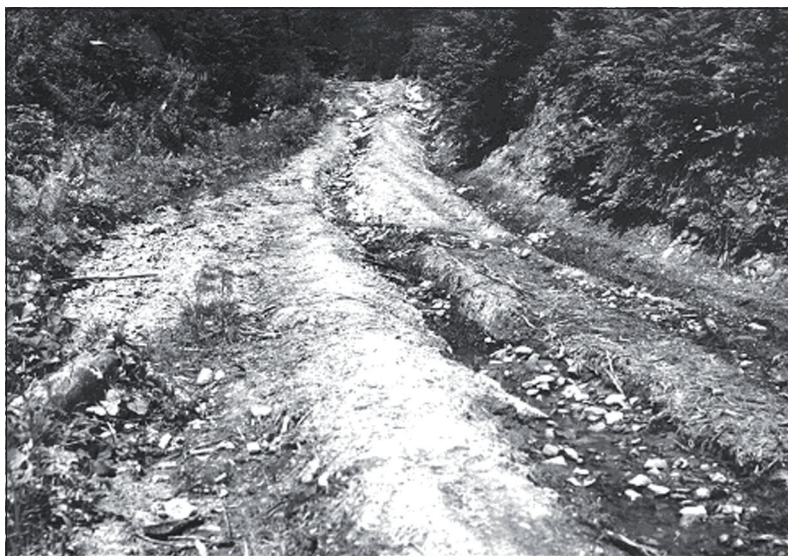
Phot. 4. The tracks left by tractors lead to the fine material outwash (phot. by L. Buzek)
