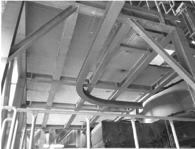
Fig. 1. An example of realization of a curve on plane hoist beam in a industrial plant (photo: author)
