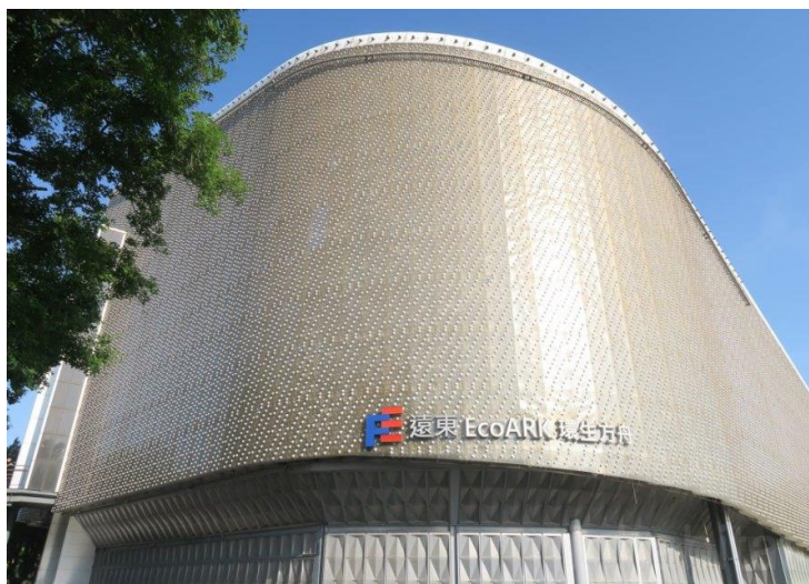
Fig. 5. EcoARK recycled plastic bottle building in Taipei.
