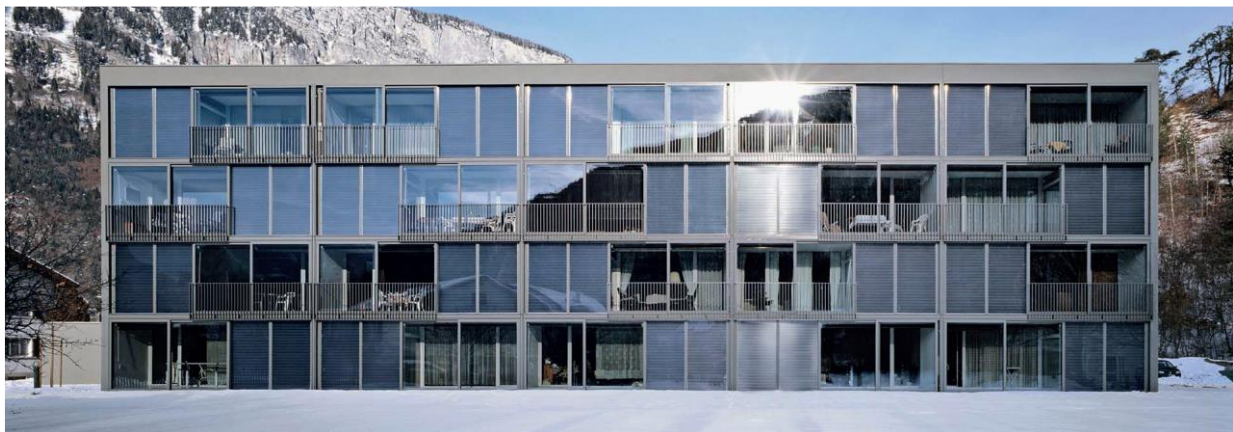
Fig. 10. Latent heat storing glass, phase change material (PCM), GLASSXcrystal. Zurich, Switzerland.
