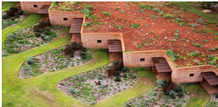
Fig. 6. Eco Houses with walls made of rammed earth
