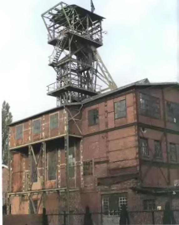
The shaft was transformed into an abyssal well, from which at the depth of 110 meters, throughout a gap with a diameter of 4,3 meters, a drinkable water is excavated from triads layer. In the set of the shaft, a brick building of shaft top with a turret, electric hoist machine from the year 1922 by Siemens and a traditional one, a 22 meter turret of the shaft with a grating construction with a viewing terrace remained in a very good condition.
