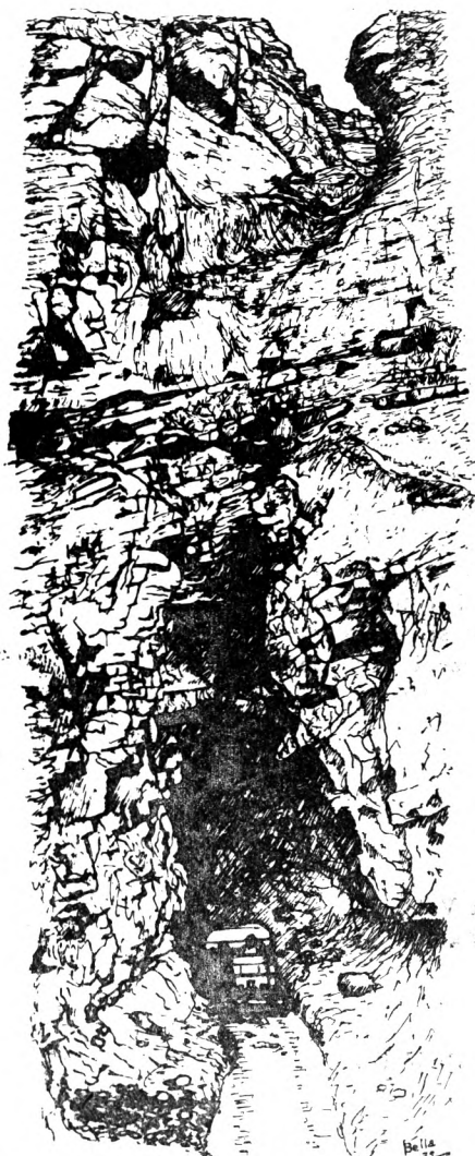
Fig. 6. Excavating a clay filling in a cave with bulldozer
